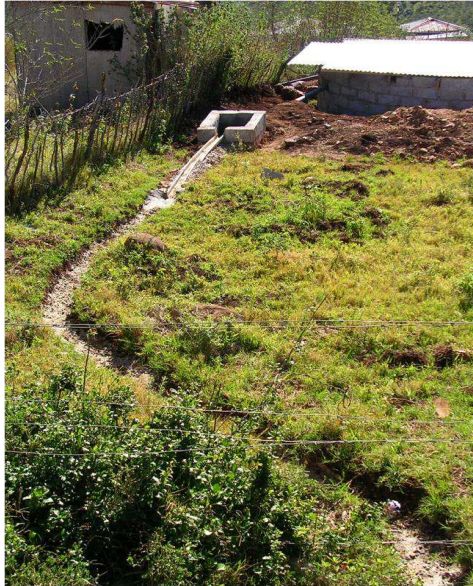
Diversion furrow leading to a catchpit
